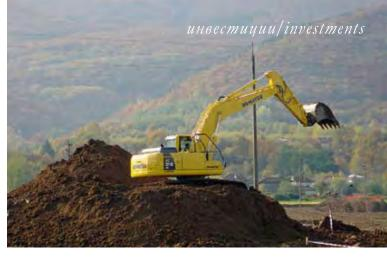
Cleaning out of these ditches and establishing new ones was a priority before major construction could commence. Since Peter Harradine's first visit in October the clearing of the vegetation has been completed and the stripping of the topsoil from the site has begun. We couldn't do a lot the last months because of the had weather. The site is also very challenging due to the high ground water table combined with the clay soil conditions.
