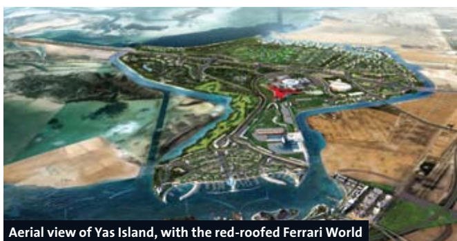
Aerial view of Yas Island, with the red-roofed Ferrari World
