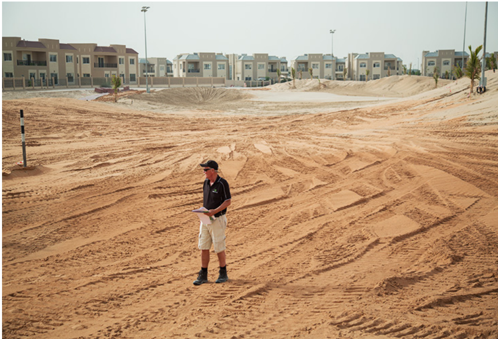
Principal designer Peter Harradine surveys progress, here on the approach to the 1st green.
